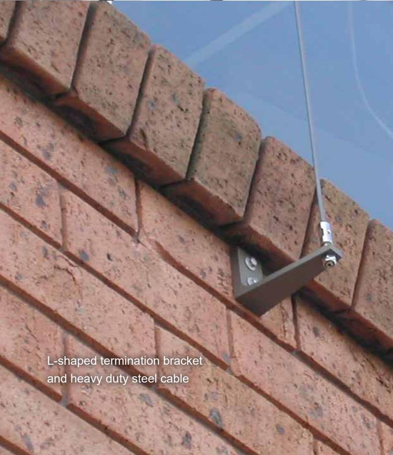
L-shaped termination bracket and heavy duty steel cable
