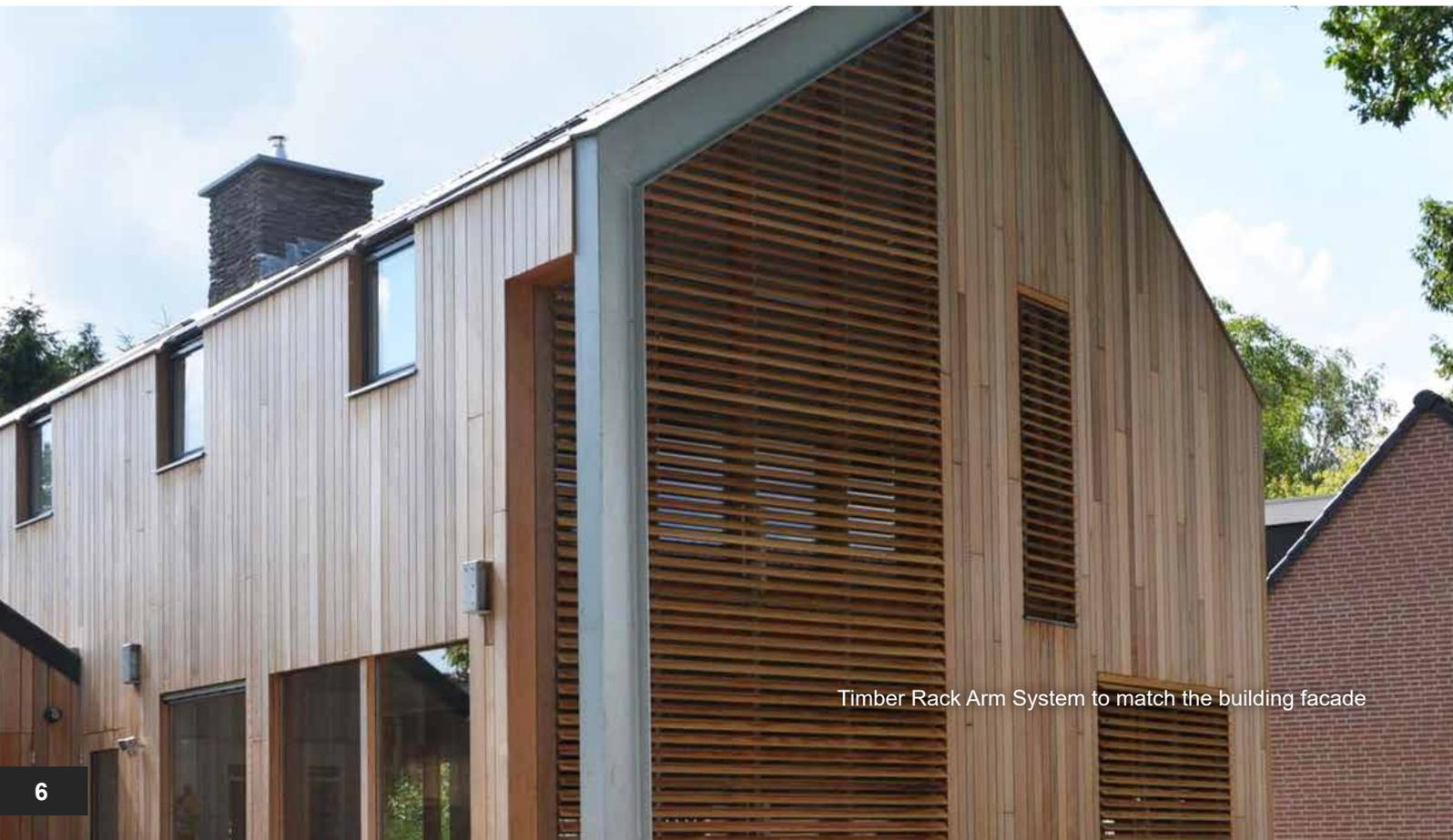
Timber Rack Arm System to match the building facade
